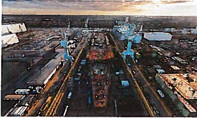
USS John F. Kennedy (CVN-79) taking shape in HII Newport News Shipbuilding Dry Dock 12 in April 2018. (Photo: HII)
